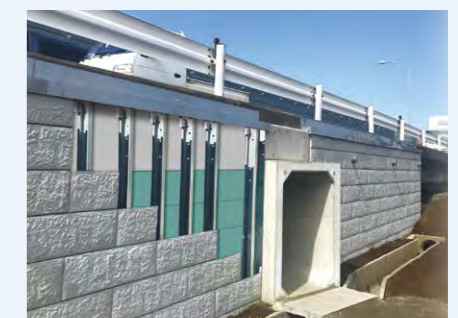
Foam Support Construction Method registered with NETIS.
